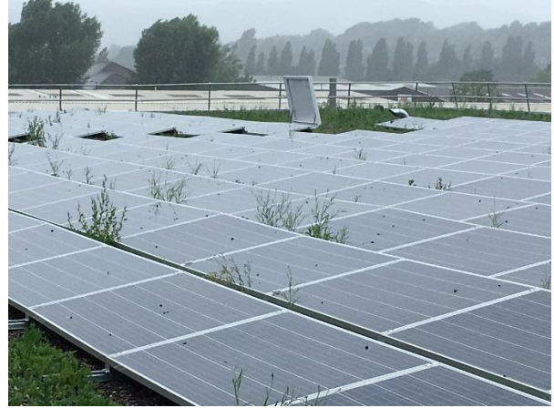
Green roof and solar panels
